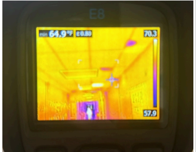
3-3-26 Floor 1 HALLWAY MD
