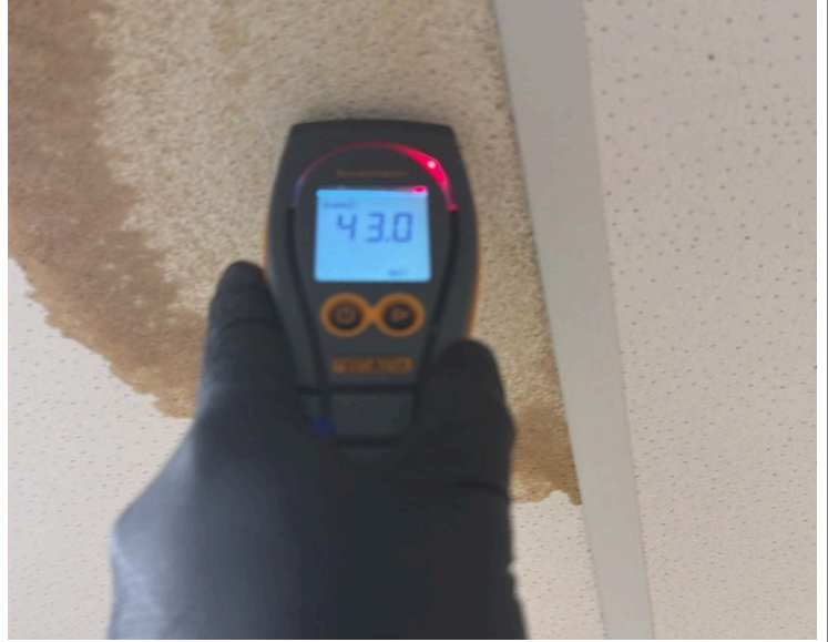
3-3-26 Floor 2 HALLWAY MD
