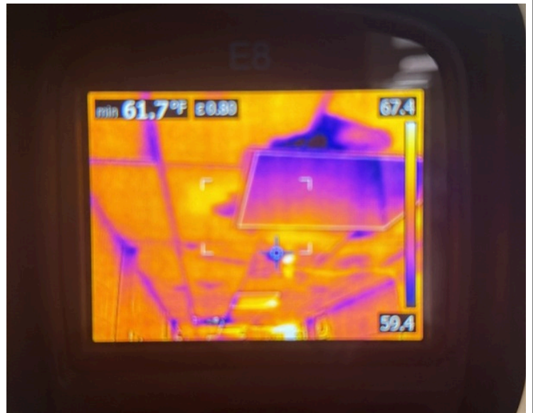
3-3-26 Floor 1 HALLWAY MD
