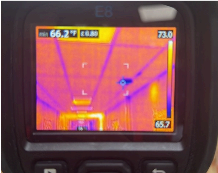
3-3-26 Floor 1 HALLWAY MD
