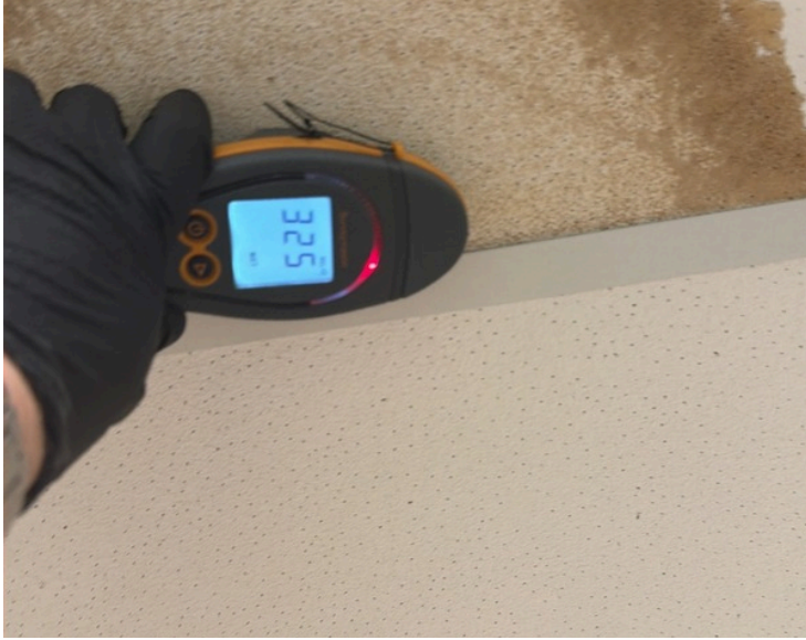
3-3-26 Floor 2 HALLWAY MD
