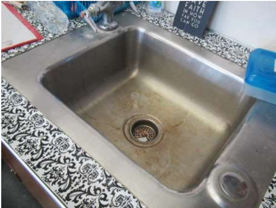
Sink countertop repaired with contact paper
